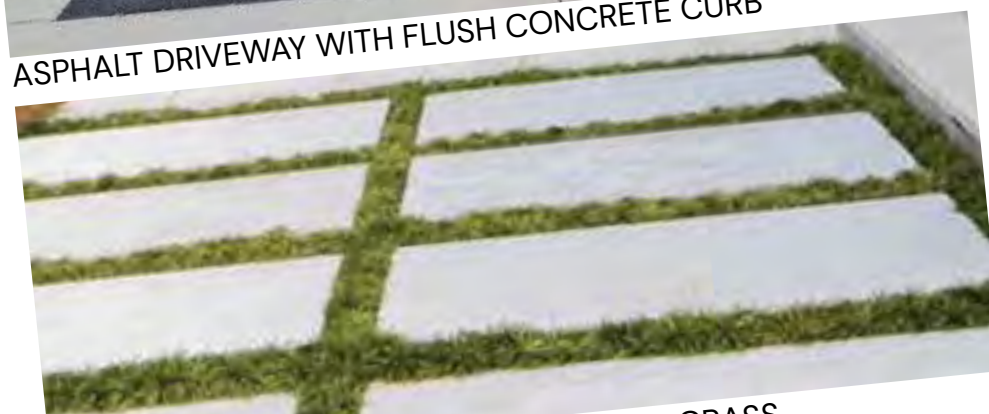
RECTANGULAR CONCRETE PAVERS SET IN GRASS
