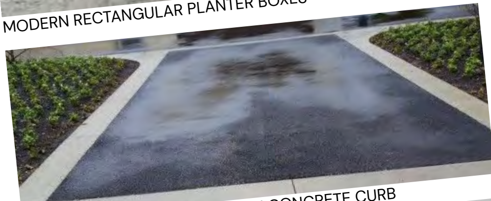
ASPHALT DRIVEWAY WITH FLUSH CONCRETE CURB
